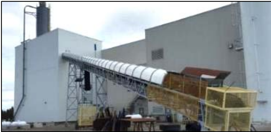
FIGURE 17.5 BUCKO BACKFILL PLANT
