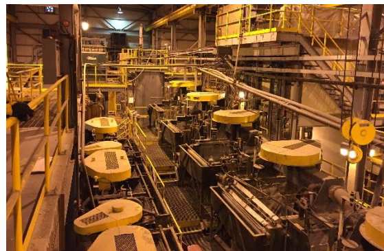
Existing Flotation Circuit
