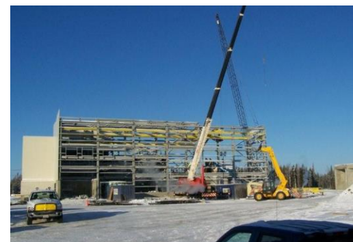
Construction of Mill Building (2008)
