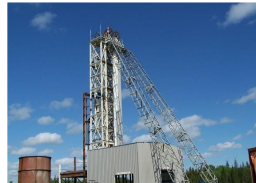
Construction of Headframe (2008)
